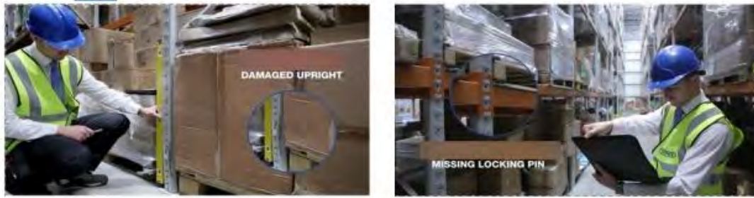
Fig 6.1.8 Inspection of Work area and Equipment
